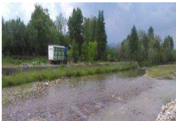
Figure 8. Reinforced concrete river bank, near Pietroșani – Bădești bridge
