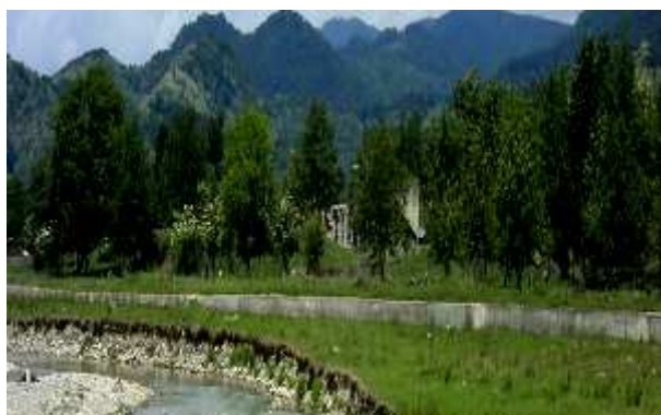
Figure 6. Reinforced concrete river bank, Domnești
