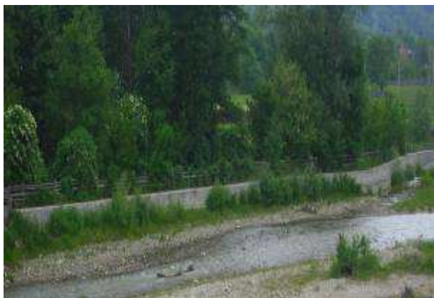
Figure 7. Concrete shores, Coșești
