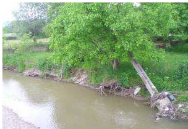
Figure 10a. Erosion, right river bank, Coșești
