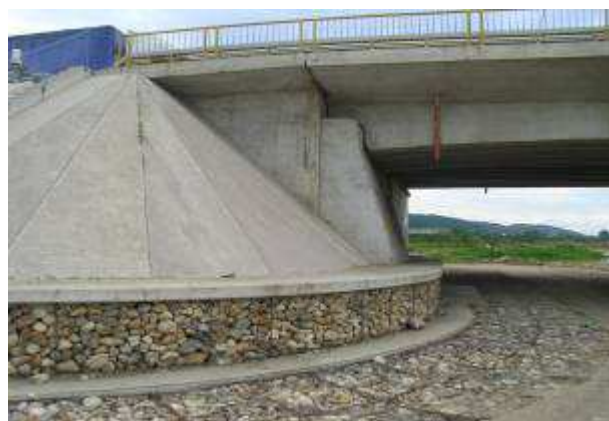
Figure 9 a, b. Protection of the banks with gabions (a) and concrete (b) for the bridge, Purcăreni, E 574
