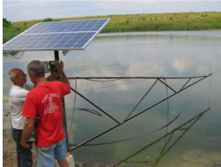
Installing the solar water pump www.muskingumswcd.org
